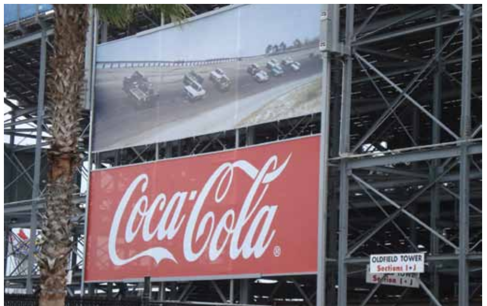
Completed BannerRail™ System, Daytona International Speedway (Daytona Beach, FL)
